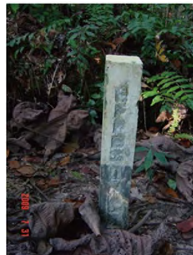
Figure T13-2 Example of stake which is resistant to disturbance (a concrete stake)
